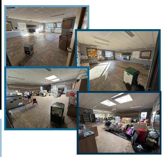
Following the Great Flood of '24, we have been spending a bit of time on the start of the repairs. The rooms have now been emptied of water damaged furniture and all floor coverings have been removed.
